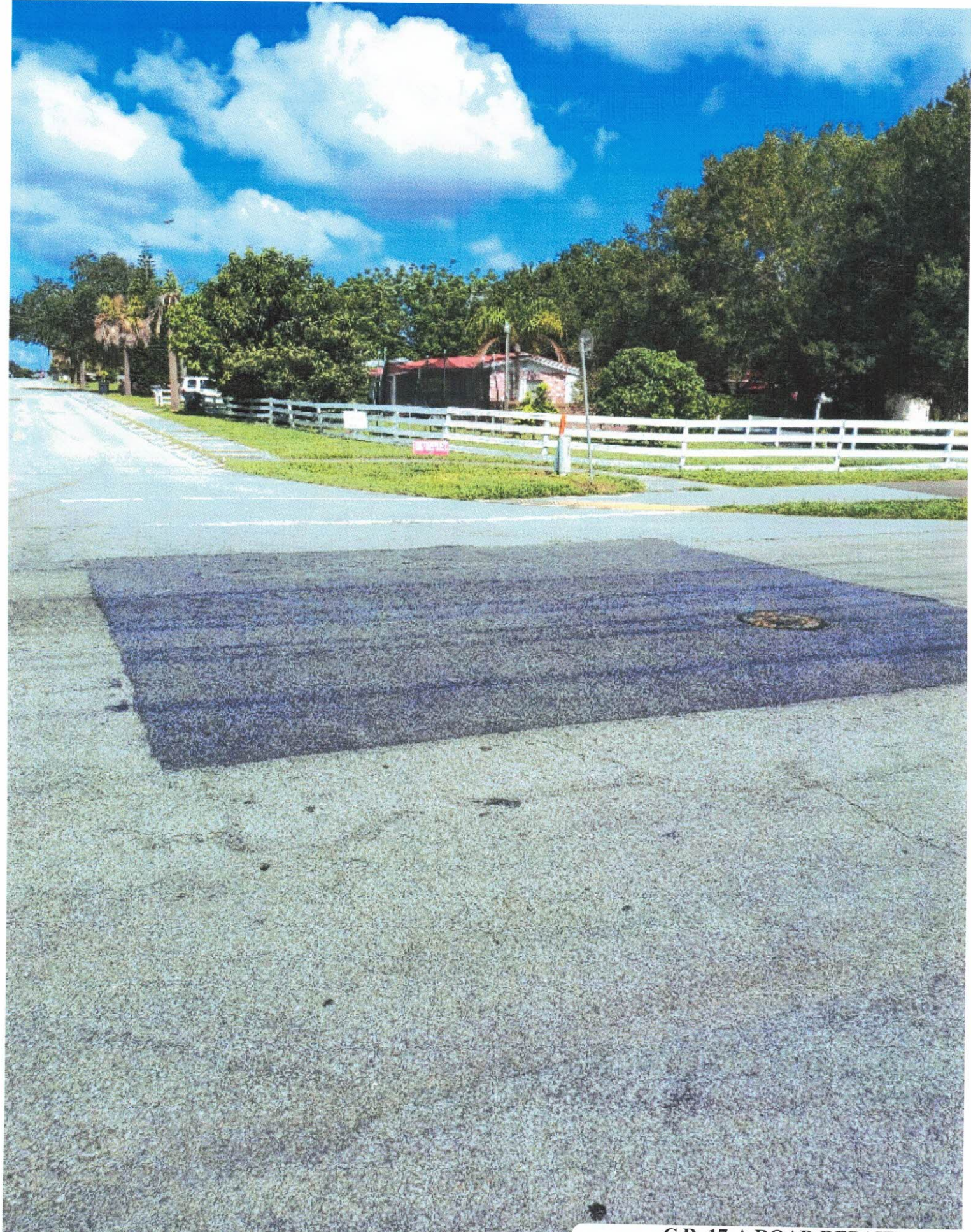
C.R. 17-A ROAD REPAIR DUE TO MANHOLE LEAK
